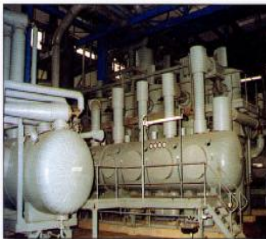
11-stage flash evaporation plant/十一效闪蒸装置
