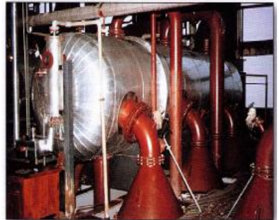
Evaporator and heaters/蒸发器和加热器
