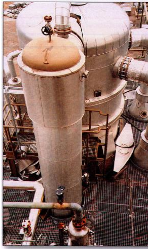
Melting crystallizer with exterior heaters and condenser/ 帶有外部加热器和冷凝器的焙烧装置
